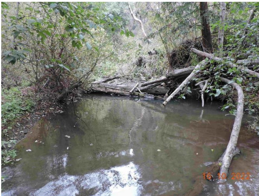
Photo 6. Looking upstream. Formerly deep pool largely filled with sediment except immediately upstream, downstream, and under the partial logjam.
