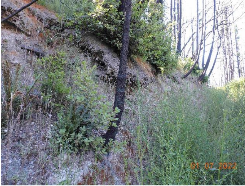
Photo 123. Bypass road, mile=2.85++. Upslope roots of tanbark oak (upper middle in photo) with dead trunk able to hold cut bank soil in place through winters of 2020-2021 and 2021-2022.
